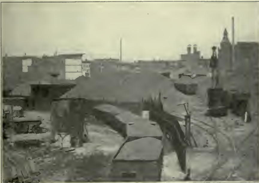
FIG. 40. STORED MATERIALS, A SOURCE OF DUST. View showing the handling of coal, August 21, 1914. In the handling of coal in the various coal yards of the city, dust is liberated, particularly when the handling is done with a locomotive crane from piles of dry coal.
